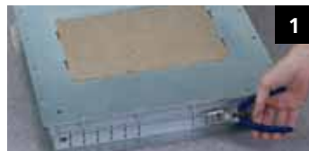
Cut the trunking entries
