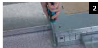
Insert the trunking and screw to floor
